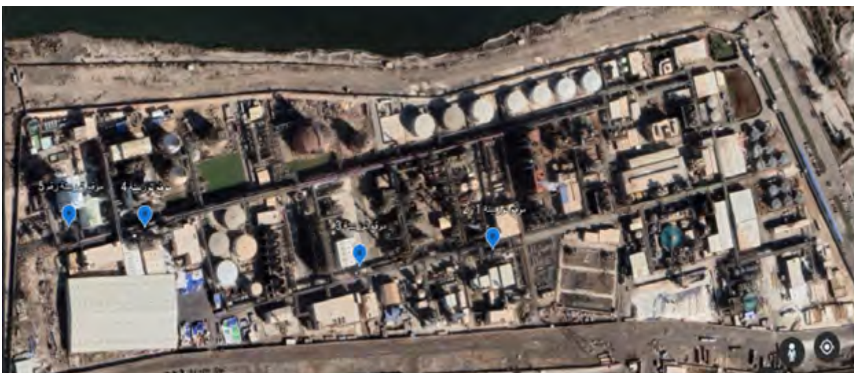
Figure 24 Location of turbines within the TCI Sanmar plant complex
